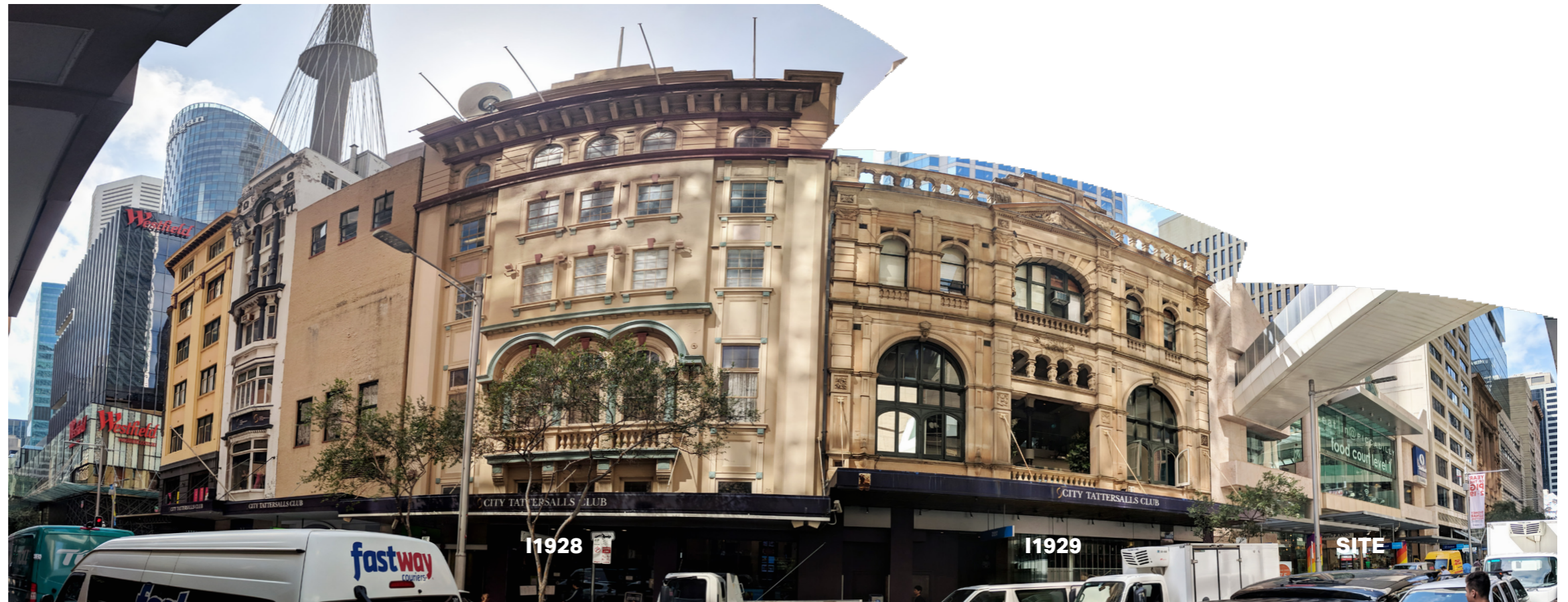
Existing view 1 - Pitt Street existing streetscape view demonstrating the adjoining street frontage heights alignment.
