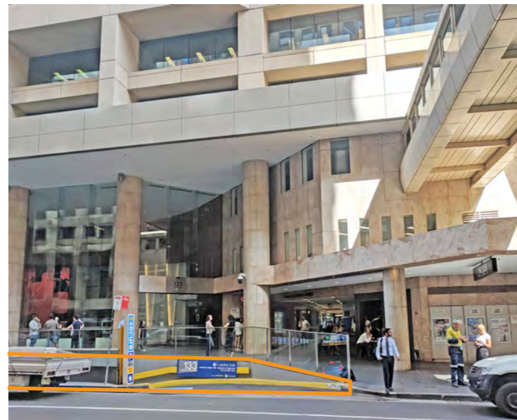
Existing View 1 - Vehicular ramp entry from Castlereagh Street.
