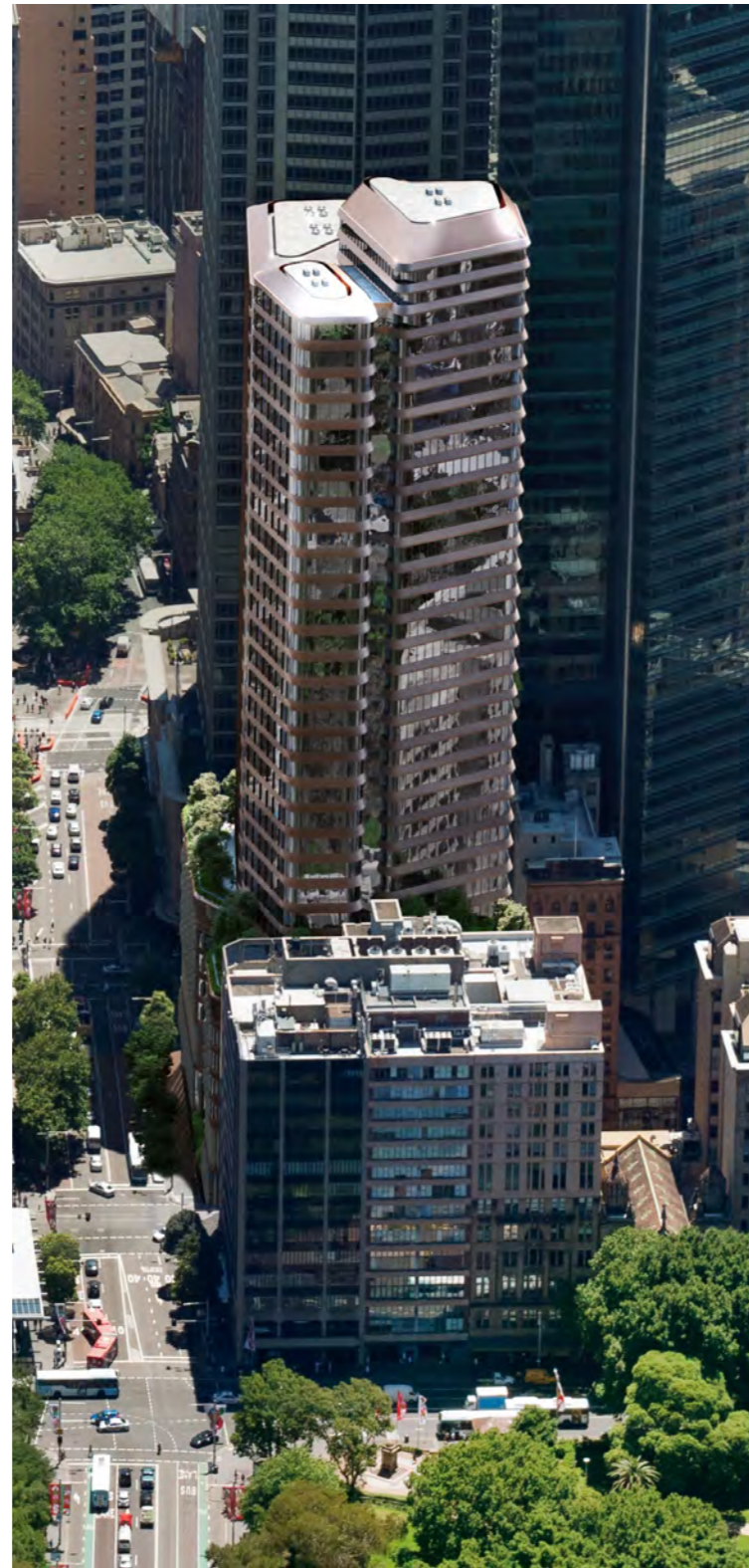
Proposal 1 - Aerial view of PSN OSD. Image source: Foster and Partners, 2020 (from DPIE Major Projects Portal)
